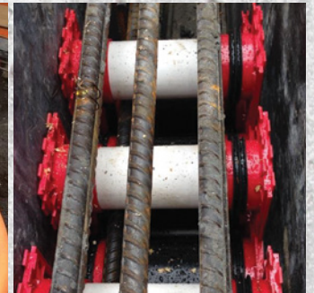
HSI150 & HSI90 wall inserts mounted in formwork
