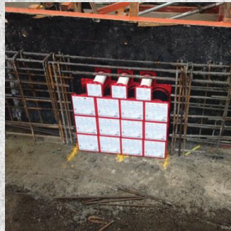
HSI150 & HSI90 wall inserts mounted in formwork
