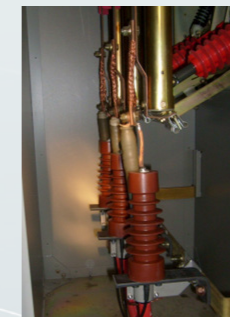
24kV Voltage Sensor installed in switchgear application
